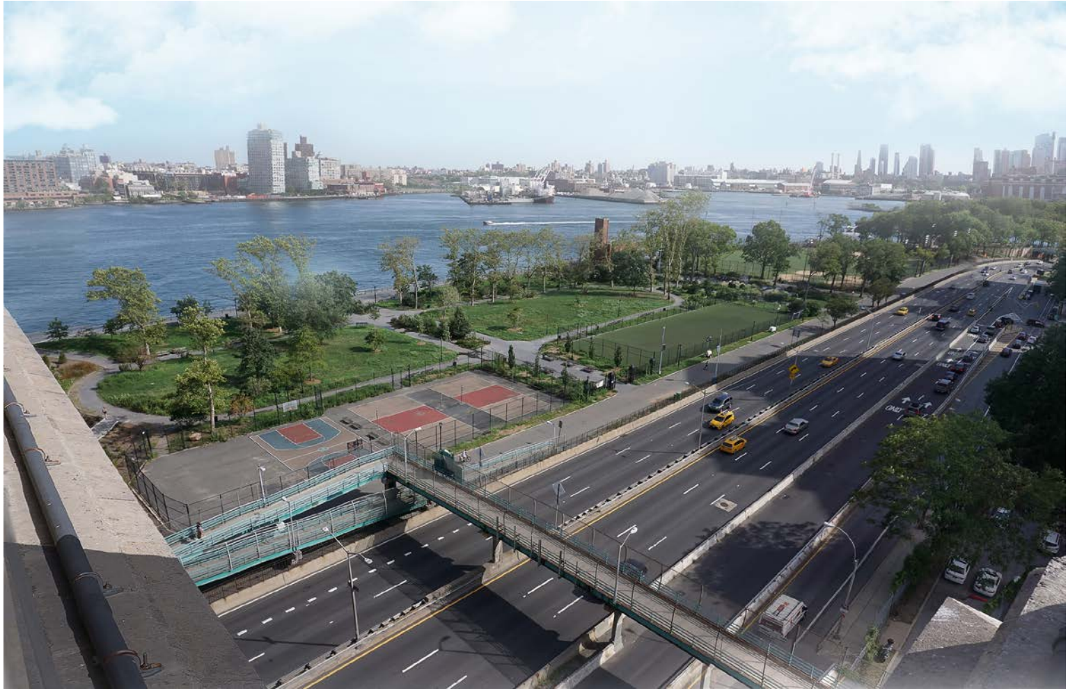
Existing Delancey Street Bridge crossing FDR Drive into East River Park
